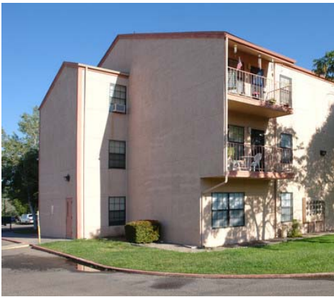
Rio Vista Apartments, Pre-Renovation
